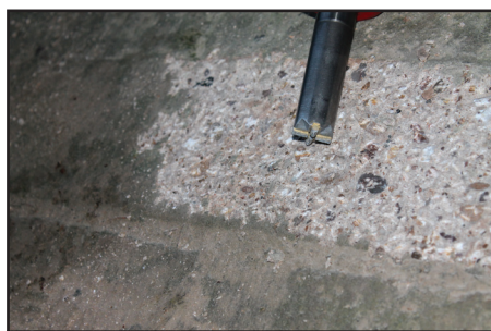
ROUGHENING CONCRETE
