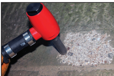
REDUCING LEVELS ON CONCRETE
