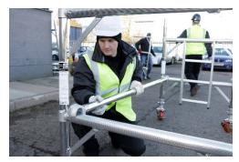
Fit another horizontal brace on the ladder side of the frames face down onto the 1st rung.
