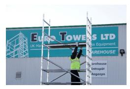
11. Fit the trapdoor platform 4 rungs above the one you are standing on. **Note:** There must always be 2 rungs clear above any platform so you can fit safe guardrail braces.
