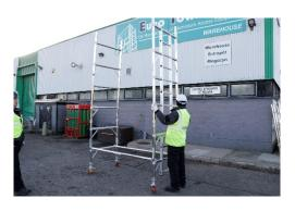
4. Fit the next set of frames onto the base, ladder frames run continuously. Note: see kitting page for frame lists.
