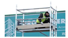
13. Fit the toeboard clips to the rung next to the corners of the platforms and then fit the toeboards as shown. **Note:** Any gap between the platform board and toeboard must not exceed 25mm.
