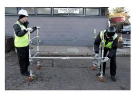
2. Fit one horizontal brace on the plain side of the frames to the vertical of the frames above the 1<sup>st</sup> rung connecting the 2 frames together.
