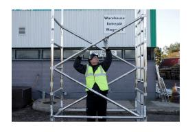
5. Add 4 diagonal braces from the  $1^{st}$  to  $3^{rd}$  and  $3^{rd}$  to  $5^{th}$  rungs as shown, level the tower using a spirit level as a guide.
